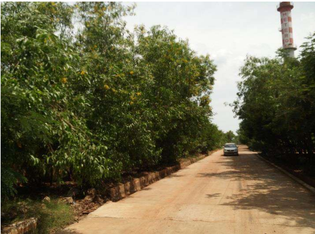
Fig. 1.16: RCC Road connected to Boilers with Green Belt
