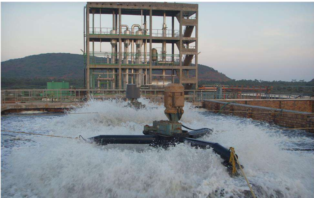
Fig. 1.12: Aeration in the effluent treatment process
