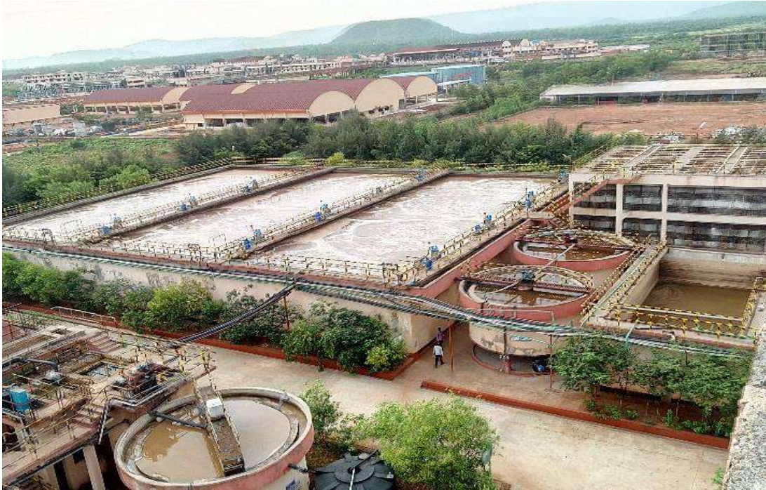
Fig. 1.9: Biological system for LTDS & Condensate of MEE & ATFD
