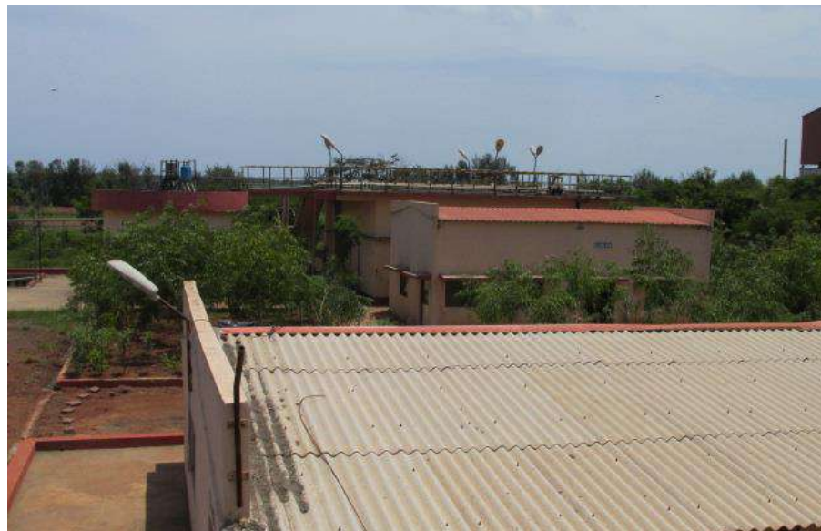
Fig. 1.4: Sewage Treatment Plant (STP)
