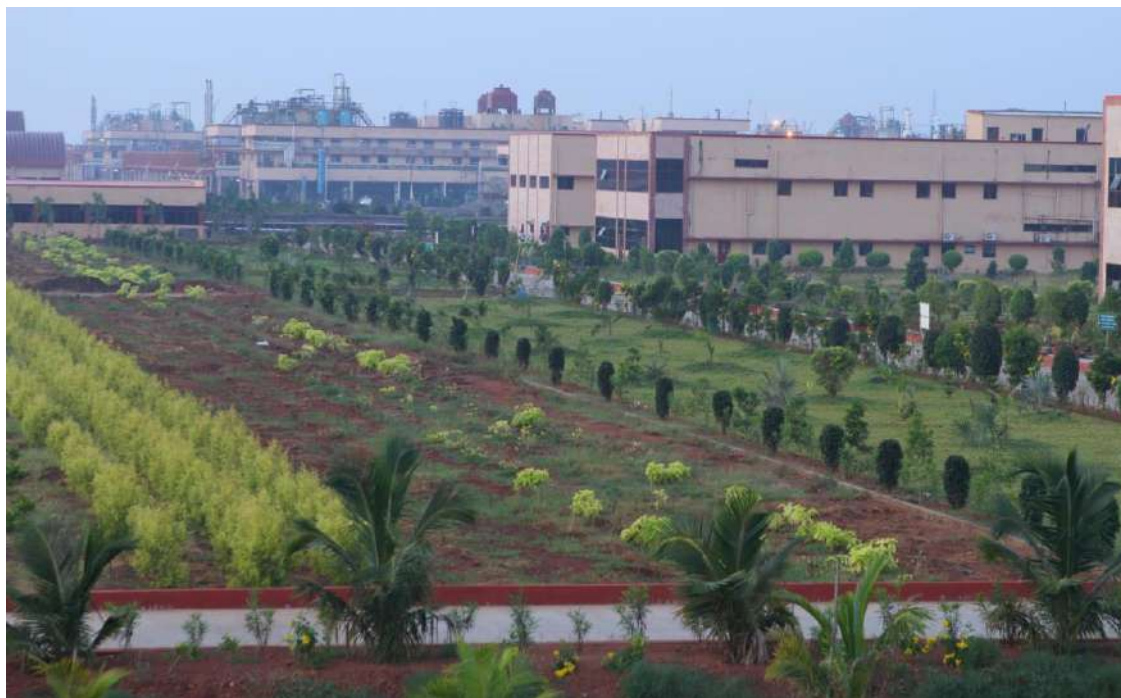
Fig. 1.13: Green Belt inside the factory
