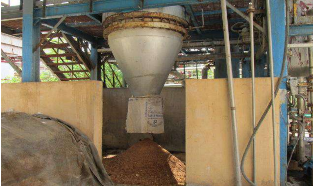
Fig. 1.7: ATFD Connected to MEE I & II
